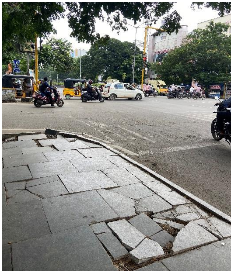
Figure 36 : Existing crosswalk at Anna Nagar area, Chennai.
